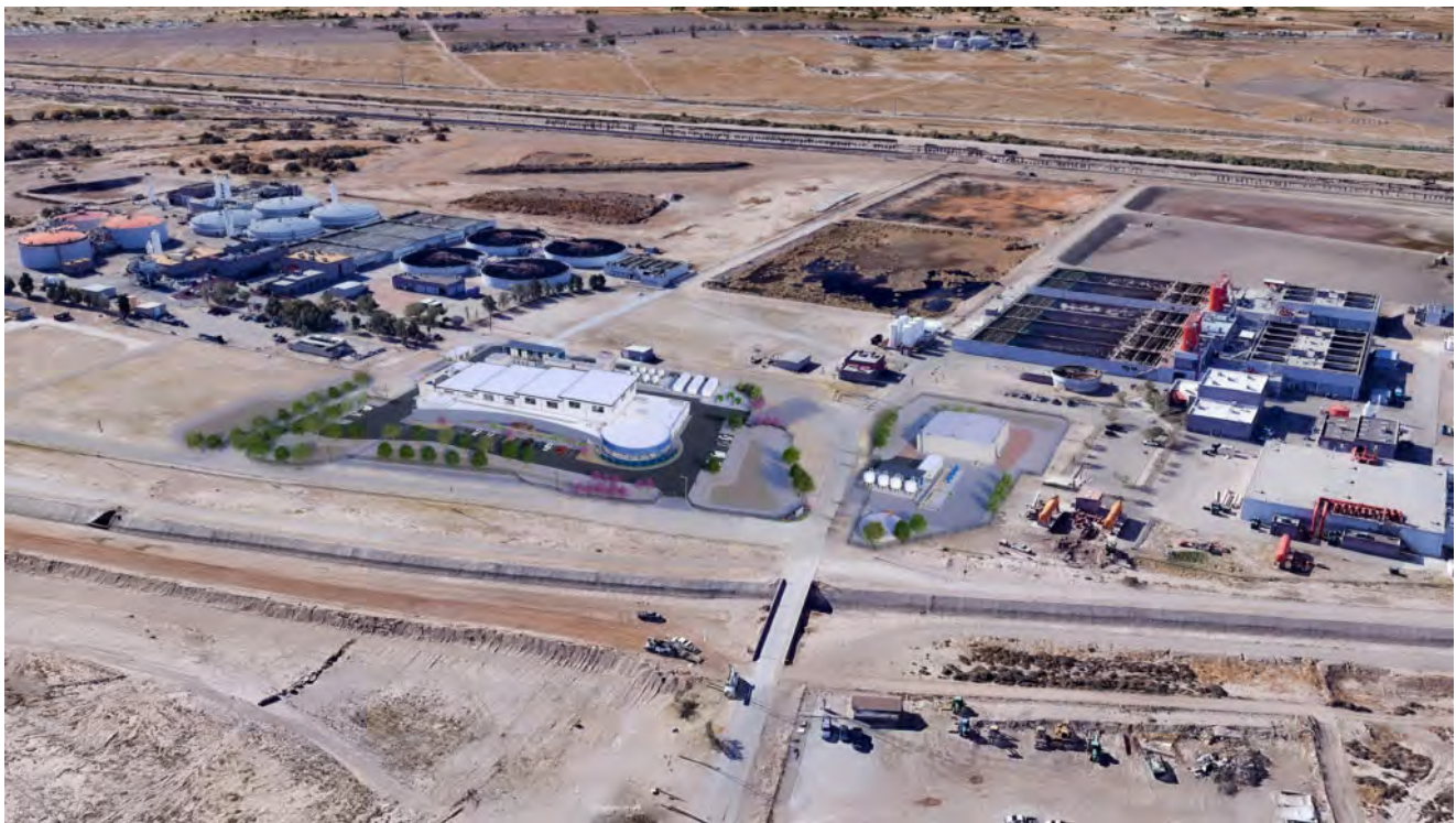
A rendering of the Pure Water Center, which broke ground on Feb. 27 and is expected to be operational by 2028. Credit: Courtesy of El Paso Water
