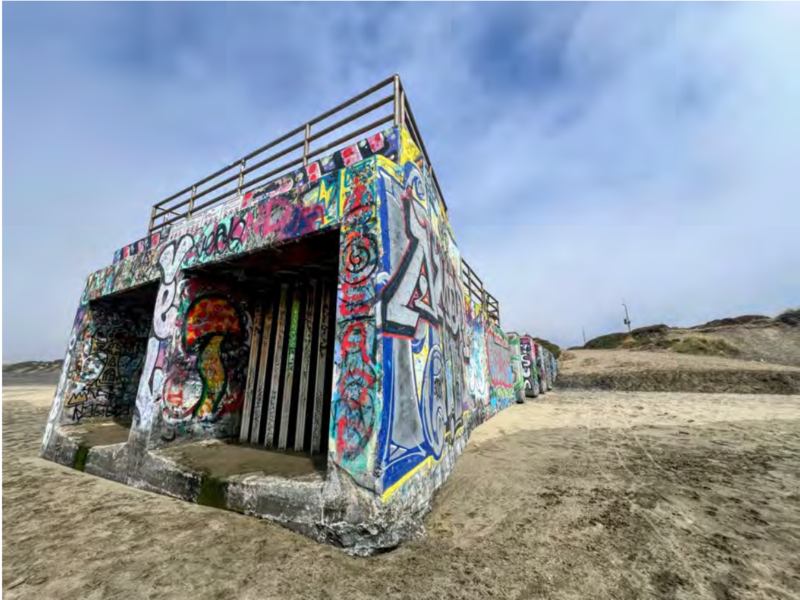
The opening of the pipes where storm and sewer water flow into the ocean during rainy season are protected by sturdy metal bars. | Jennifer Wadsworth/The Standard
