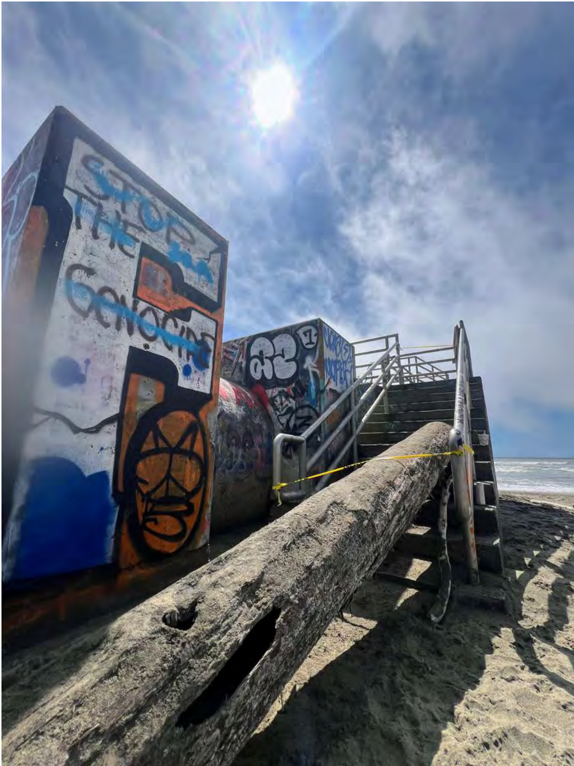
Steps lead up to a platform, where a square trap door and separate circular opening lead into the massive outflow pipes. | Jennifer Wadsworth/The Standard
