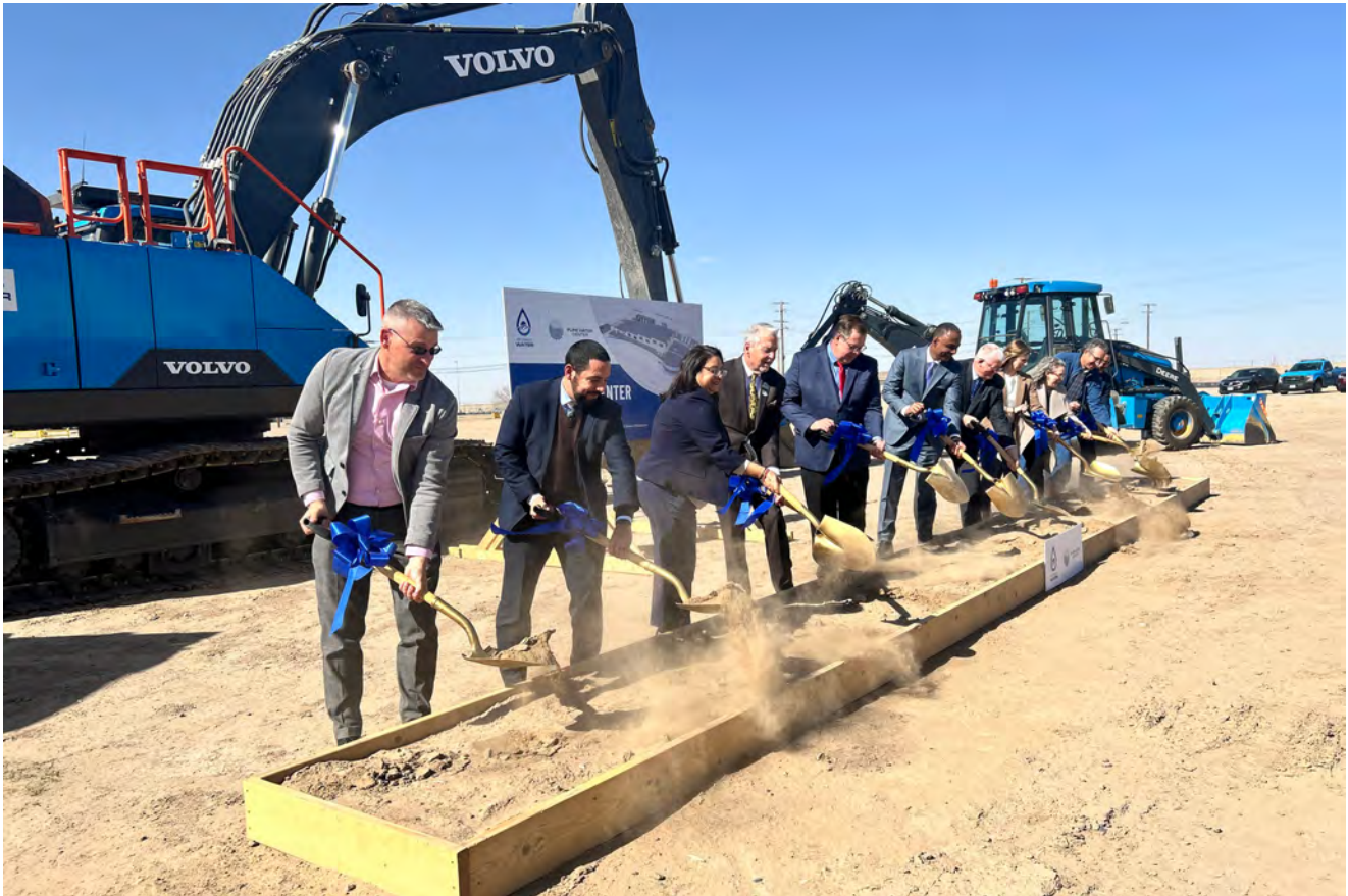
Local elected officials and water utility leadership join in the groundbreaking for the Pure Water Center. Credit: Courtesy of El Paso Water
