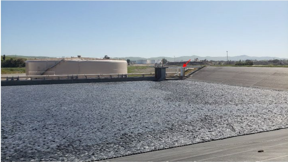
Photo 1: The west cell and one of the two new tanks in the decommissioned east cell (south half of the reservoir). The arrow points to the standpipe spillway in the west cell.
