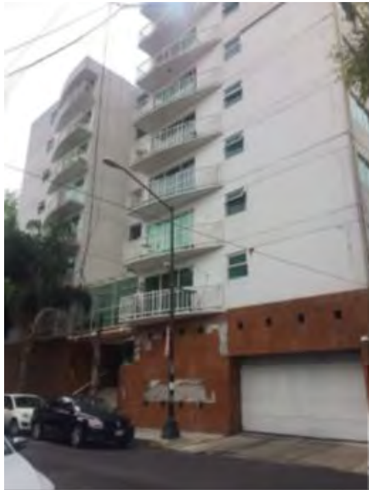
Green = No damage Ground shaking per USGS: 20.08%g
